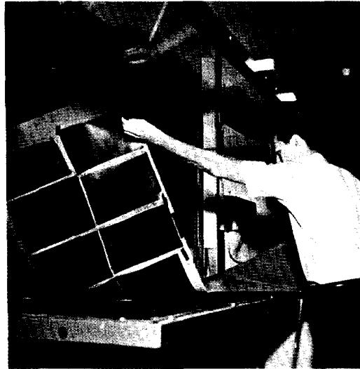
Mr. Schoon's main helper in the platemaking section is Charles Roemer. Here you see him preparing the negatives for the making of a plate. This happens to be a 16-page section of The PLAIN TRUTH . First, he carefully covers any scratches or holes there may be in the negatives with a black paint. This is called opaqueing , because what the process does is to keep light from passing through the negative wherever it is applied, making it opaque. Next, Charles lays the complete section of negatives on a frame over a light-sensitive metal plate, and locks it into position. The last picture shows the powerful arc light burning through the negative and forming an impression on the plate.
